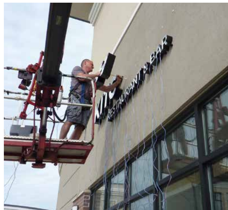
Kitchen 1883 in Anderson Towne Center
